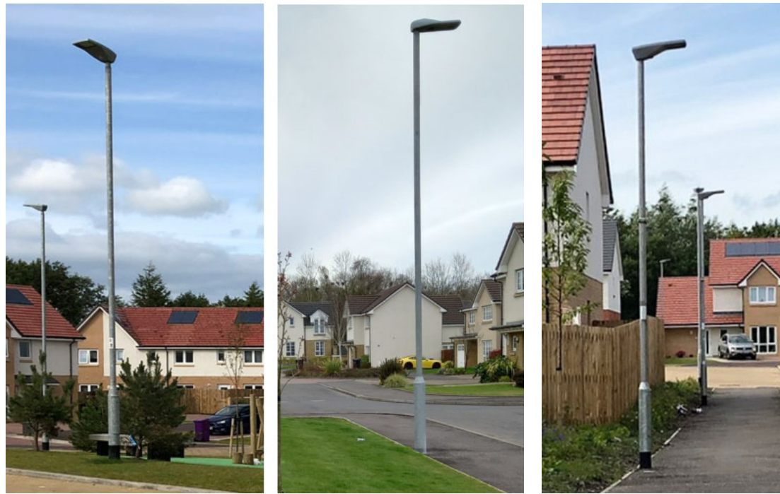
Figure 1,2 & 3 – Galvanised Finish Column Lighting with LED Lamps in Public Realm
